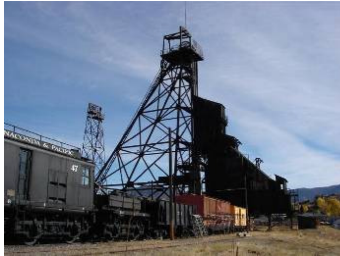
The Amselmo Mine Yard Interpretive tours and signage offer a unique look at mining technology for Butte's citizens and visitors.
