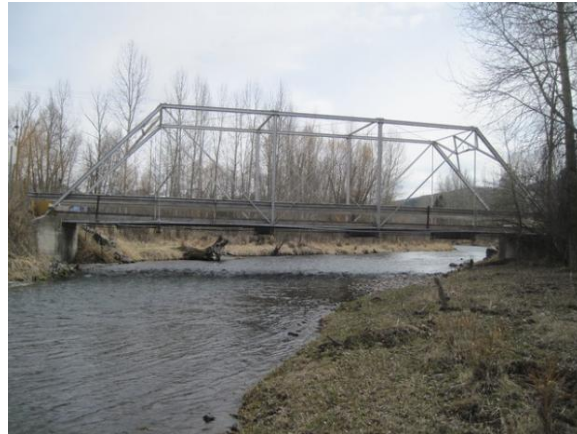
Jocko River Bridge, Lake County
