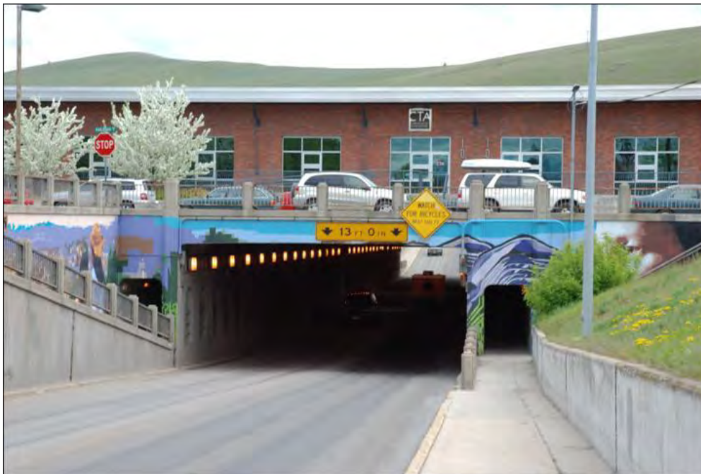
Photo 0002. Orange Street Underpass. South side. View to north.
