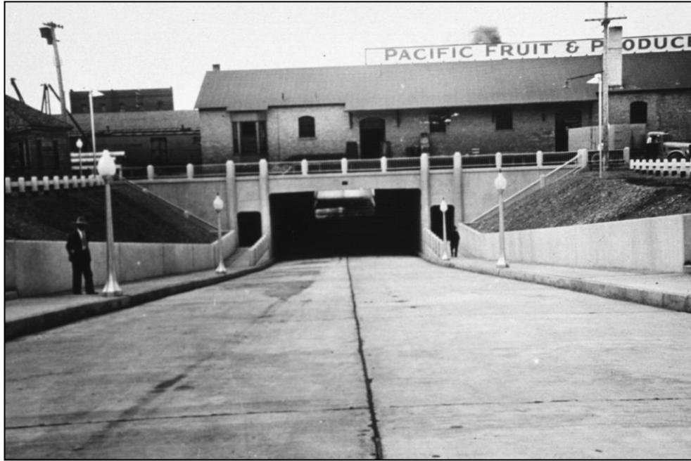
Photo 0001. Orange Street Underpass. North profile. View to the south.
