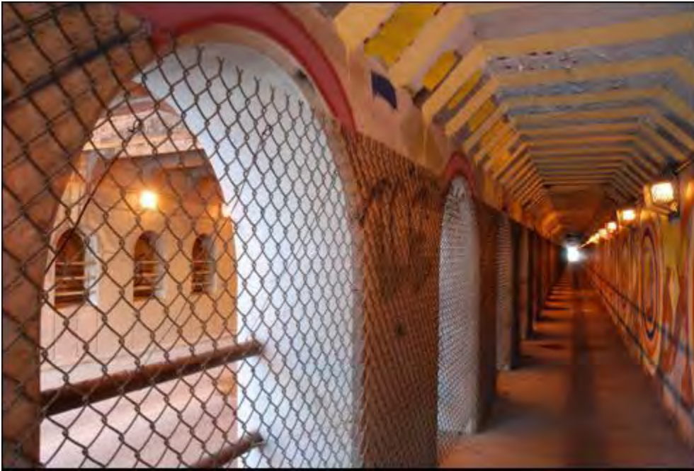
Photo 0005. Orange Street Underpass. Detail of arcade walkway. View to north.
